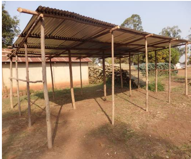
Temporary Structure for Brick Laying classes
