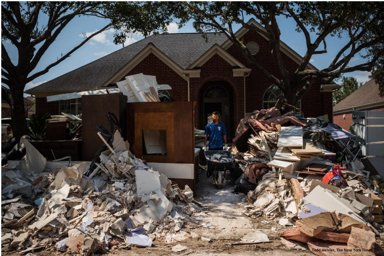
Removing debris after Hurricane Harvey
