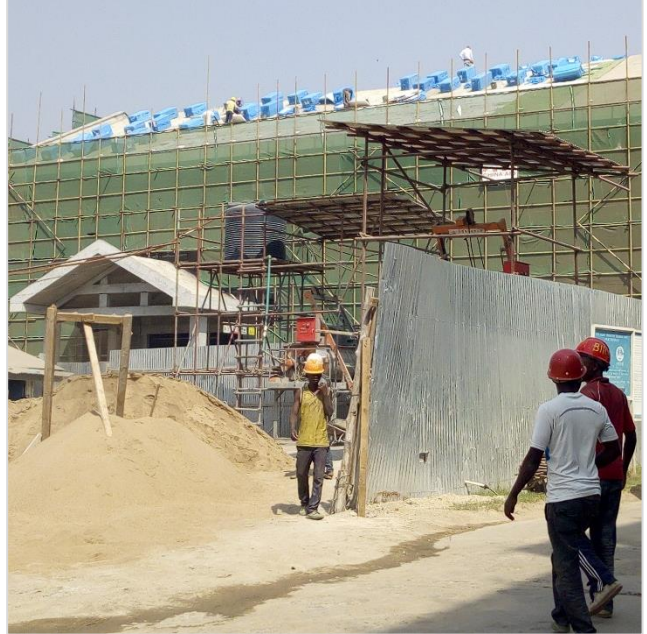
JTH's new Maternity ward in its latest stage of construction
