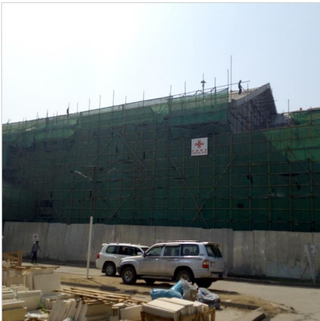
Ongoing construction progress of JTH's Outpatient department
