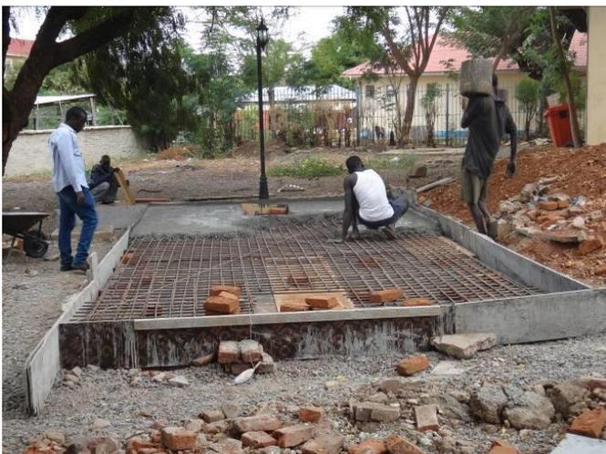
Repair of the JTH main septic tank in progress
